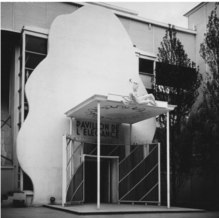
Figure 6 Pavillon de l'Elegance, Exposition Internationale des Arts et Techniques dans la Vie Moderne, 1937, photography by Dell and Wainwright, Paris, France.
